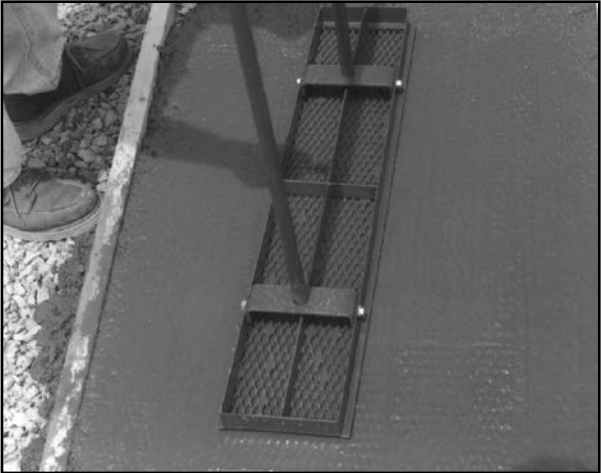
2. Lightly tamp concrete and then screed to specified grade.
