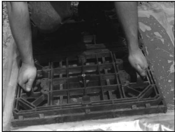
6. Imprint concrete with BossCrete™ imprinting tool.
