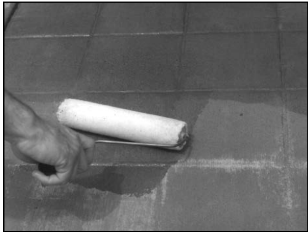
7. Apply a sealer after touch-up work is completed.
