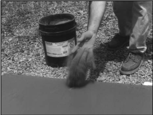
3. Once excess bleed water has dispersed, apply the first application of Bon True Color™
