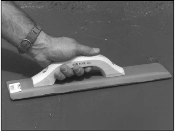
4. Use a wood or magnesium float after first application.
