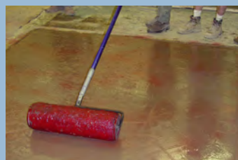
4. Add True Color™ Release and texture with roller
