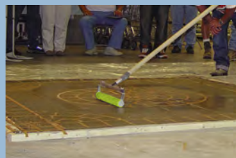
2. Embed stencil with roller
