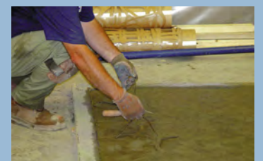
5. Remove stencils and seal
