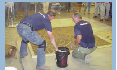
3. Add True Color™ Hardener and float concrete
